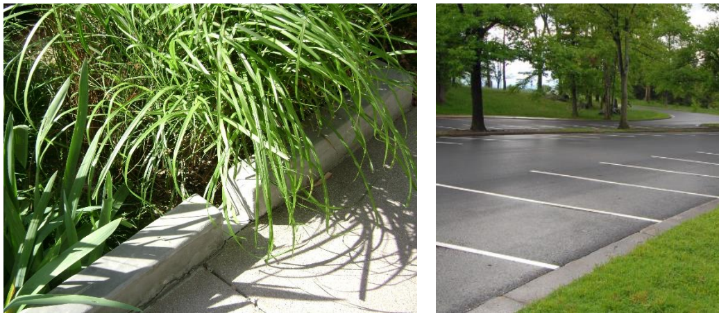
Examples of curb cuts and parking area applications allowing for water infiltration.
